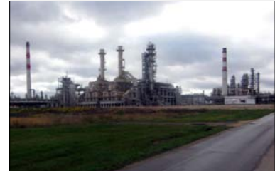
Lukoil site (600 ha) in Kstovo
